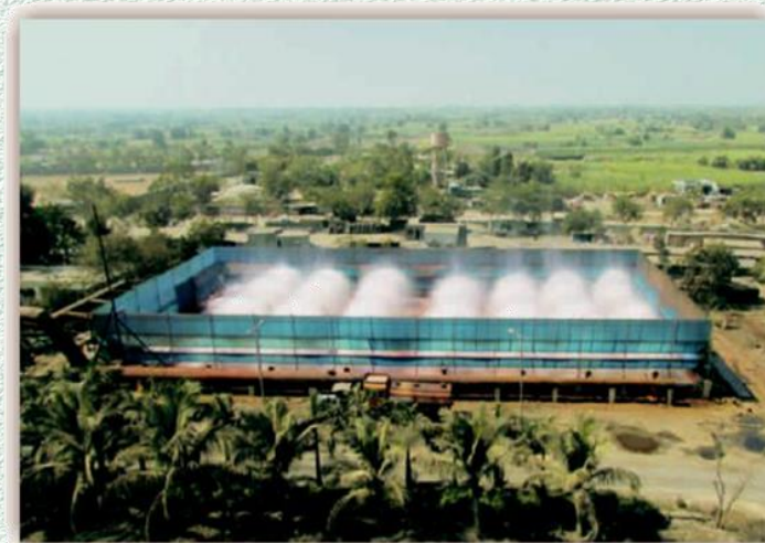
Louver Type Mist Cooling System.
